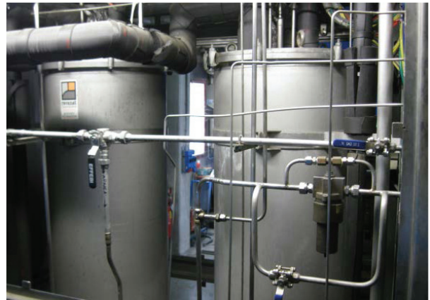
Fig. 7. LN2 purification unit
